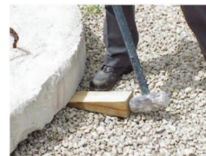
Inserting a wedge to initiate cribbing
